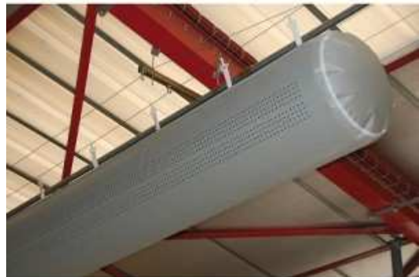
Air diffuser for distributing air uniformly
